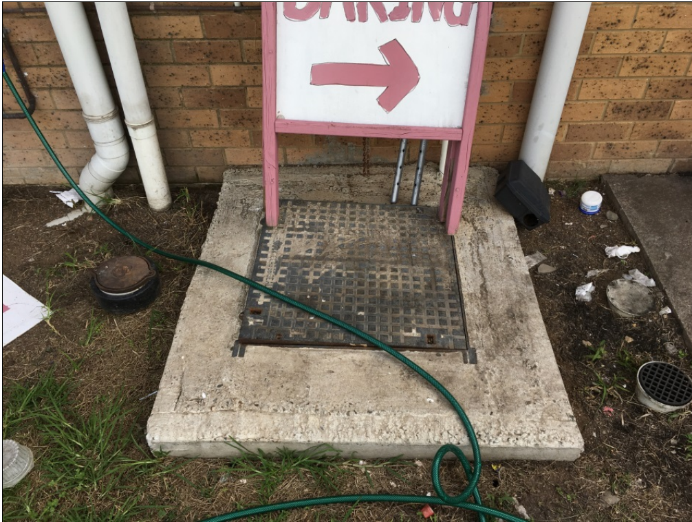
Figure 8: Lid of grease trap located at the rear of building, looking west.
